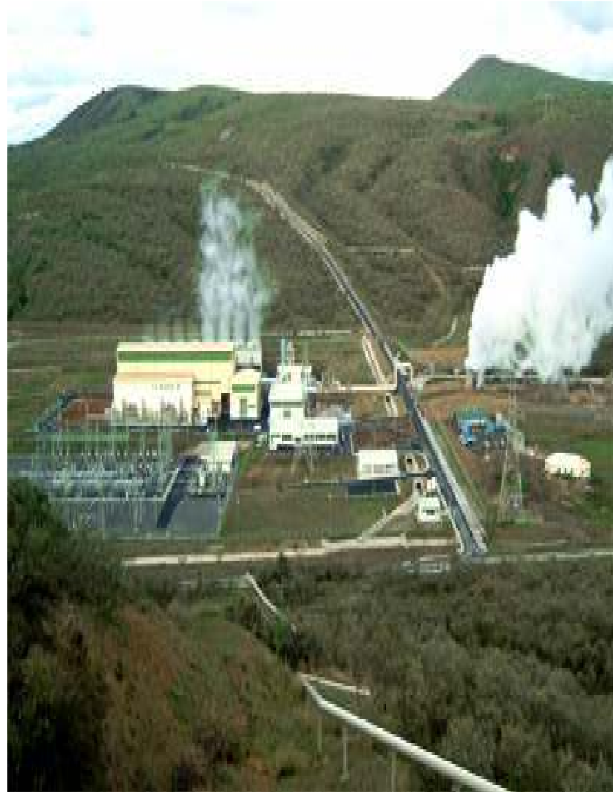
OL-KARIA GEOTHERMAL PLANT
